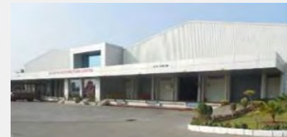
Parts Distribution Center - Pithampur
