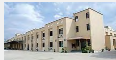
Eicher Engineering Component – Dewas
